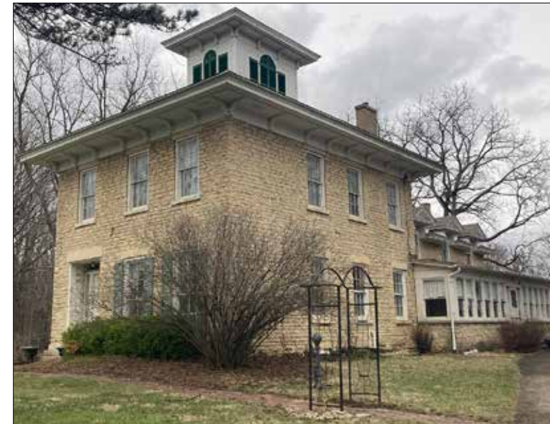
Hanchett-Bartlett Homestead's only entrance sidewalk is very narrow and has settled along the front of the house, looking northwest from the driveway. April 13, 2022
