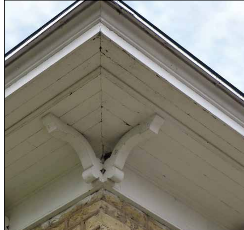
Detail of the Hanchett-Bartlett Homestead roof eave. April 13, 2022
