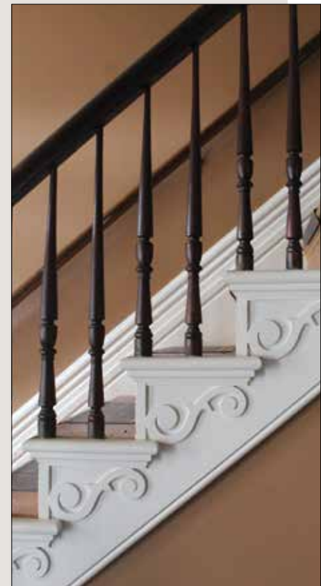
Hanchett-Bartlett Homestead interior stairway April 13, 2022
