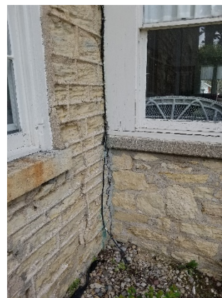
A-10: Crack at Porch, Wrong Joint Material
