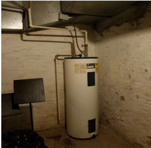
P-5: Existing domestic water heater
