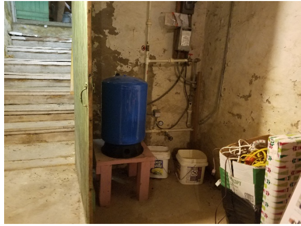
P-2: Well water service entry and pressure tank
