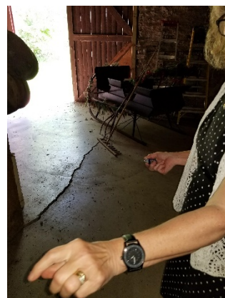
A-25: Barn Floor Crack
