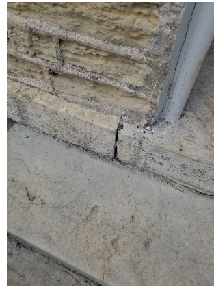
A-8: Entry Open Stone Joints
