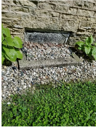
A-13: Infilled Basement Window
