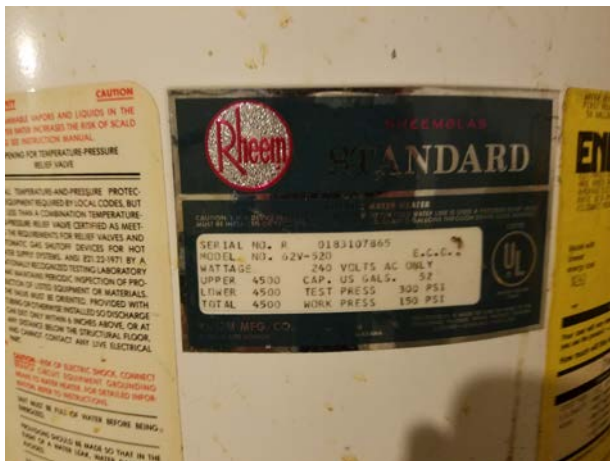
P-9: Water Heater Label - 1 st four numbers of serial number indicates date of manufacture.
