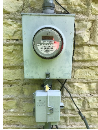
E-2: Service Meter/ Telephone NID
