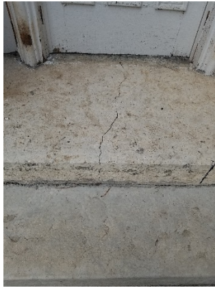
A-7: Crack at Entrance Stone
