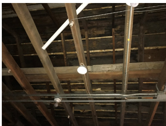
E-11: Knob and Tube Wiring
