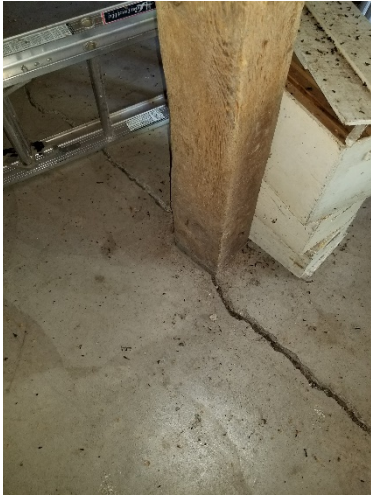
A-26: Barn Floor Crack
