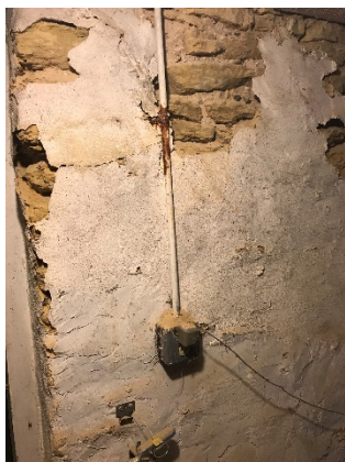
A-17: Basement Wall Peeling
